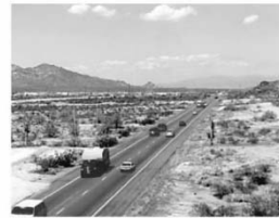
Level of Service "B"
