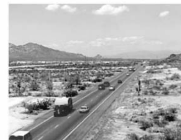
Level of Service "B"
