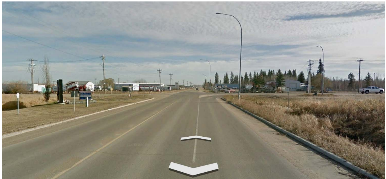
Viewing east on Hwy. 38 West towards the intersection with Hwy. 644/44 th Street. Intersection has exclusive right turn lane for turning to the south.
