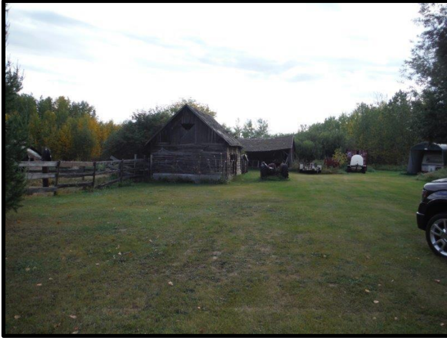
Picture 7 - Additional view of the buildings at the residence in the northwest portion of the subject site.
